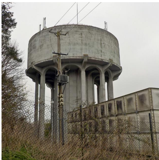
Figure 5 – Water Tank, Tank Farm
